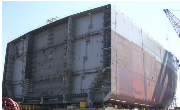
Figure (e): Fore body built on slipway
